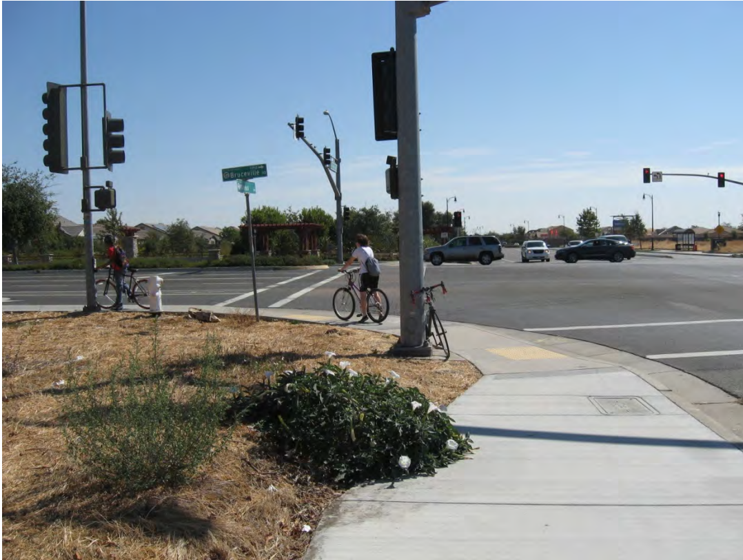
Current Situation – The trail ends at the utility driveway forcing cyclists onto the sidewalk or bike lane. For easterly travel, the sidewalk is the only option.
